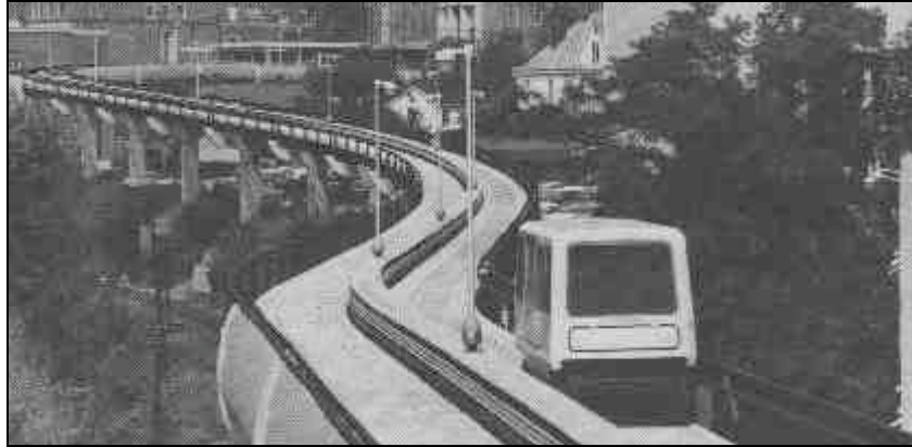
Figure 6, Two-way, elevated, heated guideway. Photo from http://faculty.washington.edu/~jbs/itrans/morg.htm .
