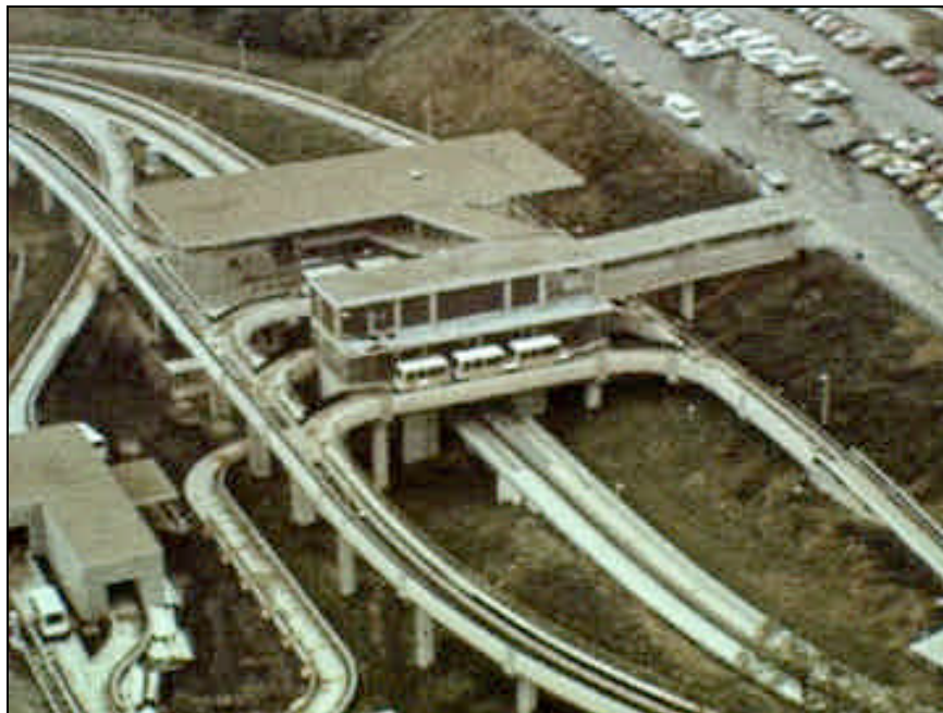
Figure 3. Engineering Station: 6 channels, bypass underneath the station, and adjacent maintenance facility. Photo from http://faculty.washington.edu/~jbs/itrans/morg.htm .
