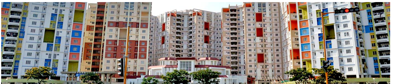
Apartment complexes in MAR (SE extension) road
