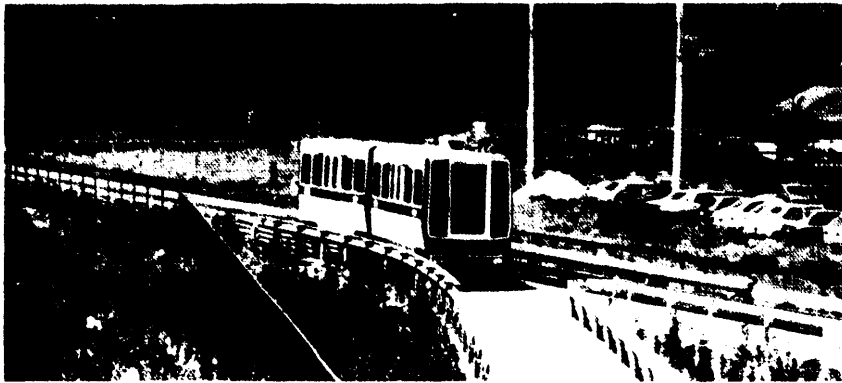
Test Track built by LTV Licensees, Niigata Engineering Co. and Sumitomo Shoji Kaisha, Ltd.
