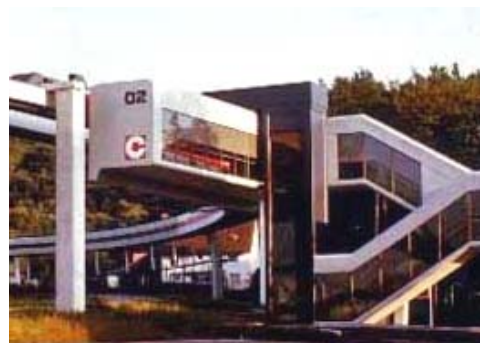
Figure 17 - Cabintaxi Test Track Station
