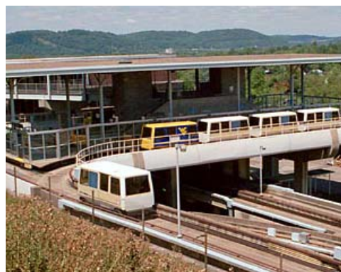
Figure 1 - Morgantown Off-line Station
